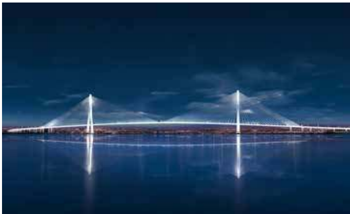
One component of the I-75 Michigan Exchange expansion project is the Gordie Howe International Bridge, which will be the longest cable-stayed bridge in North America. Image courtesy of AECOM.
